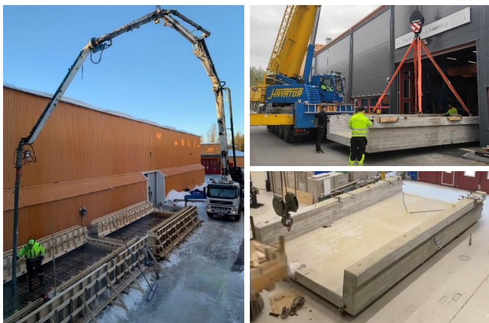
Figure 20: Casting Day for the trough bridges (left), transportation of TB1 (right, top), TB1 inside the laboratory (right, bottom).
